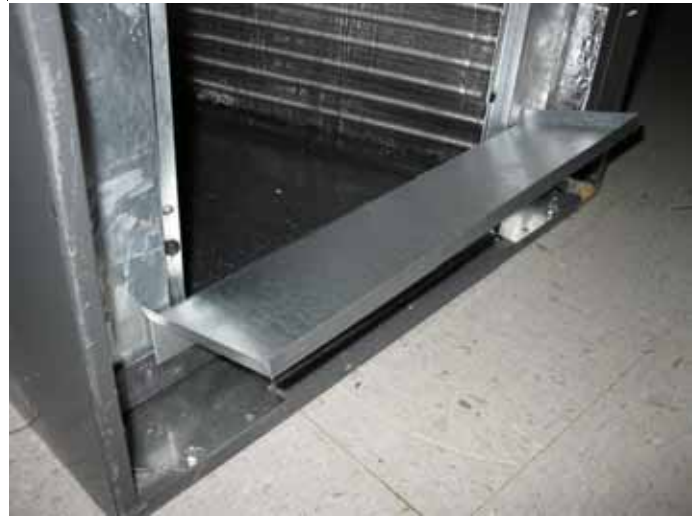
Figure 6 Horizontal Blow-Off Bracket
